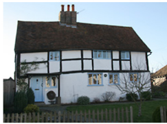
(2) Applebough Cottage 16th century timber-framed cottage of a style that is rare in Surrey
